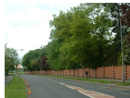
Fig. 6 Existing eastern boundary along Bishopthorpe Road
