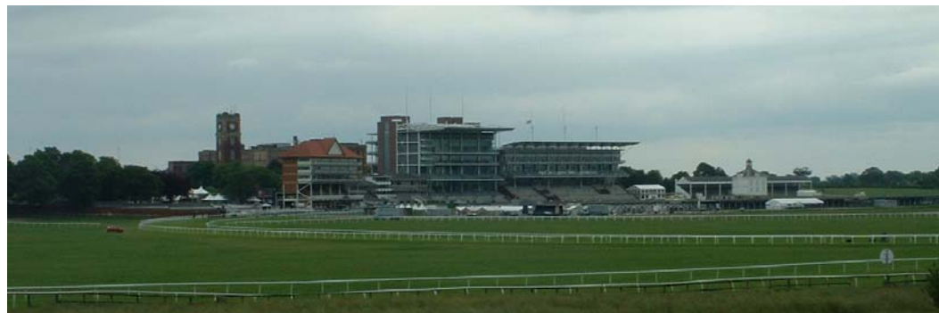
Fig. 10 Conservation Area from west
