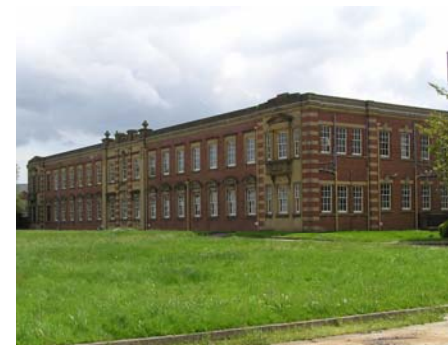
Fig. 4 Line of existing boundary along the northern elevation of Head Office
