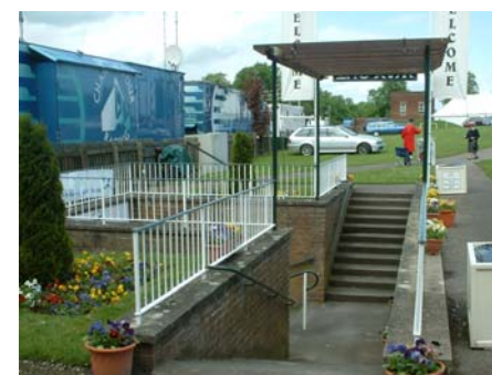
Fig. 42 Steps across Racecourse Road
