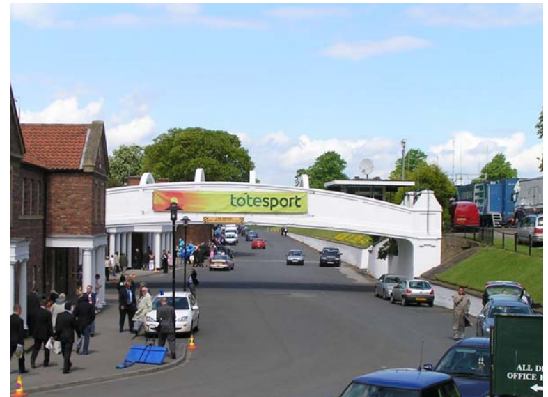
Fig. 35 Bridge link across Racecourse Road
