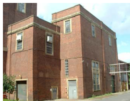
Fig. 53 Boiler and Transformer house
