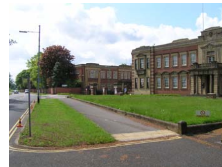
Fig. 24 View of the frontage buildings along Bishopthorpe Road
