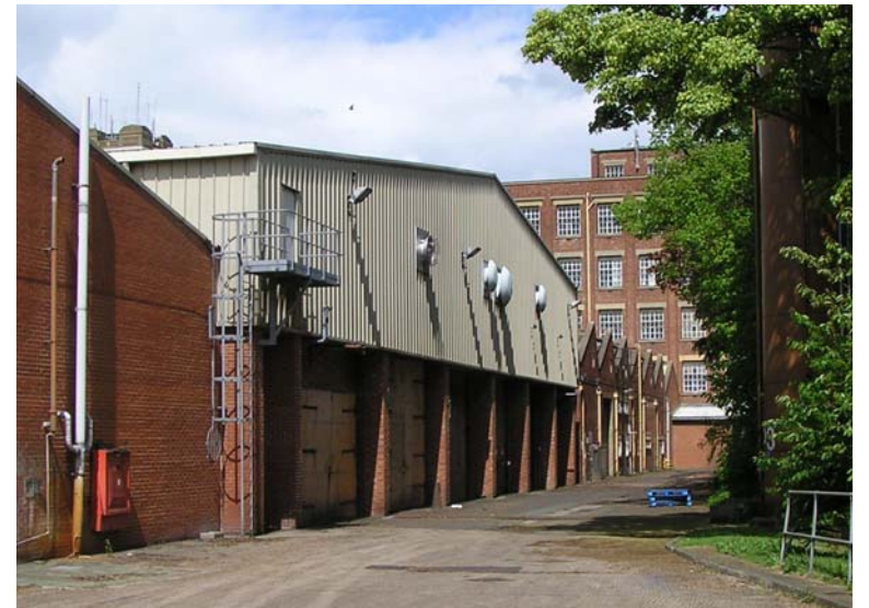
Fig. 45 View looking north-west within factory grounds
