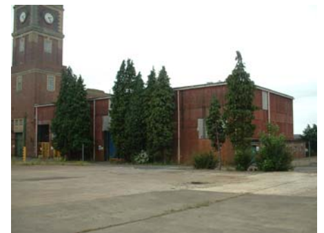
Fig. 3 Later extension to Boiler House
