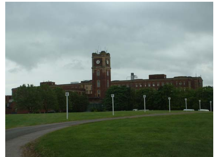
Fig. 40 View south-east across Park Pavilion Field
